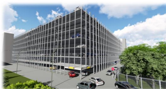
Multi-Storey Car Park 7
