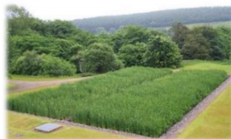
Indicative Wetland Water Treatment Facility
